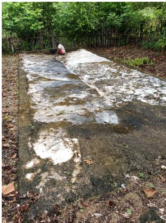
Figure 1 Water pan built over exposed Limestone Karst
